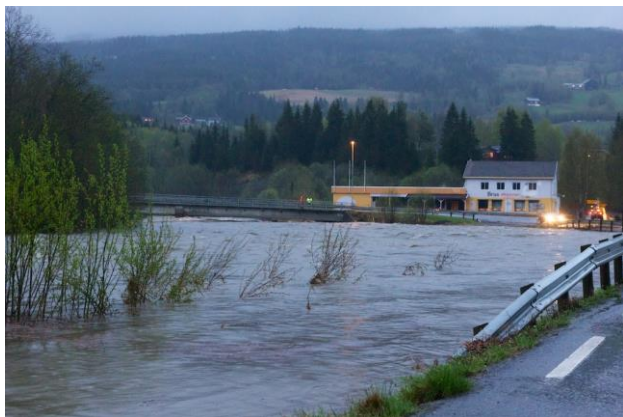
Bridge in Gausdal threatened by flood, 2013
